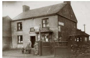
The Original Post Office
