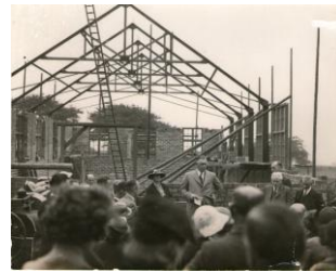
Construction of the hall
