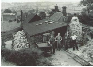
Workers outside the drying shed
